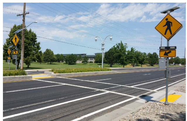
Rectangular rapid flashing beacon
