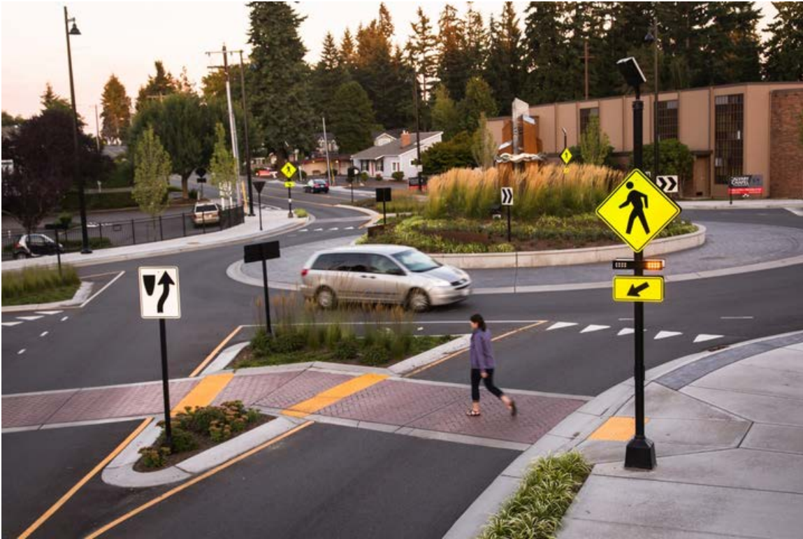
Fig. 8: An example of roundabout design, with pedestrian beacons, a lowered roundabout edge, and pedestrian islands.
