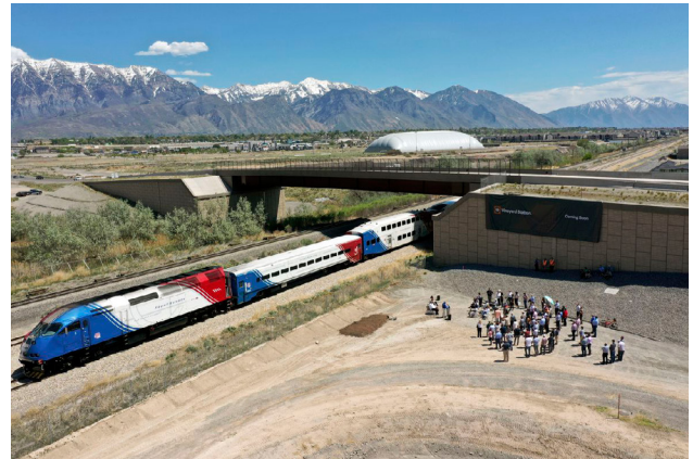
Figure 1.7 Vineyard FrontRunner Station Groundbreaking
