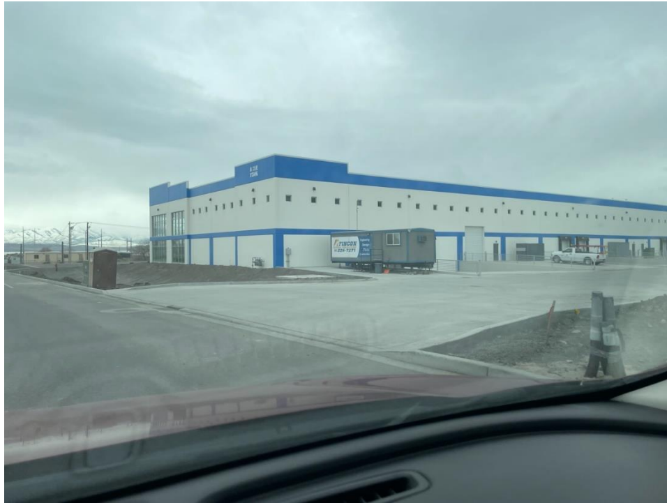
Photographs of the New Constructed Lot 05 Buildings from Tuesday, February 21, 2023,
