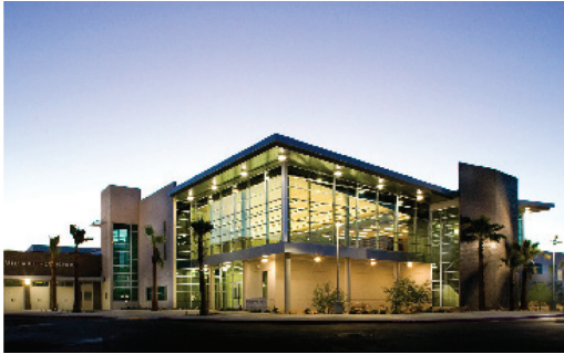
Northwest Career & Technical Academy Project included 10,000 SF Library, 6 Career focused Academies, Media Labs, teaching kitchen Owner: Clark County School District Las Vegas, NV Services Provided: Architecture & Planning *Winner of the James D. McConnel Award, Council of Educational Facility Planners International, A4LE- GTS
