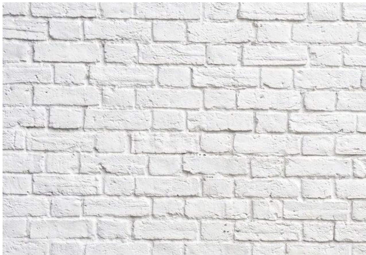
MASONRY PAINTED WITH COLOR 3
