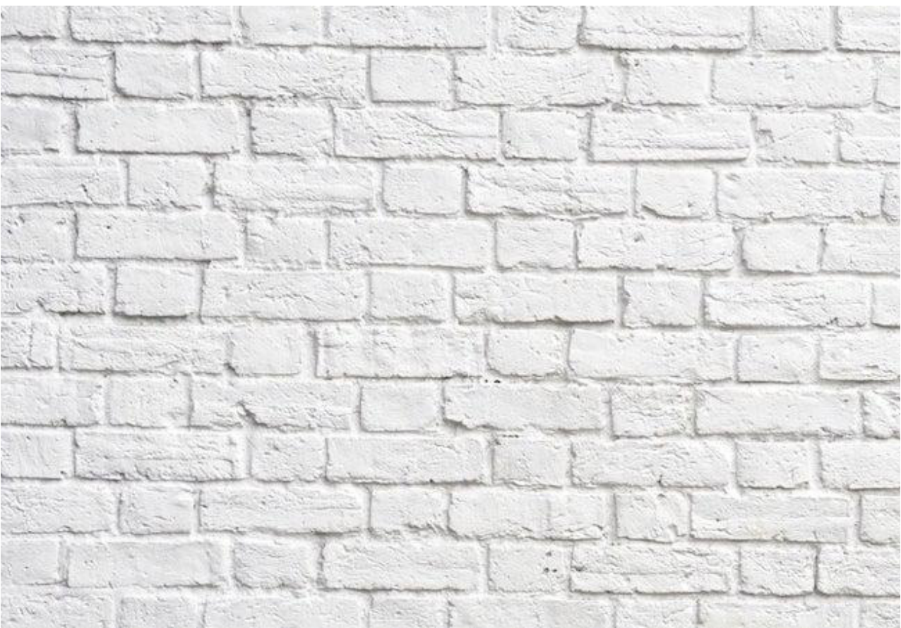
MASONRY PAINTED WITH COLOR 3
