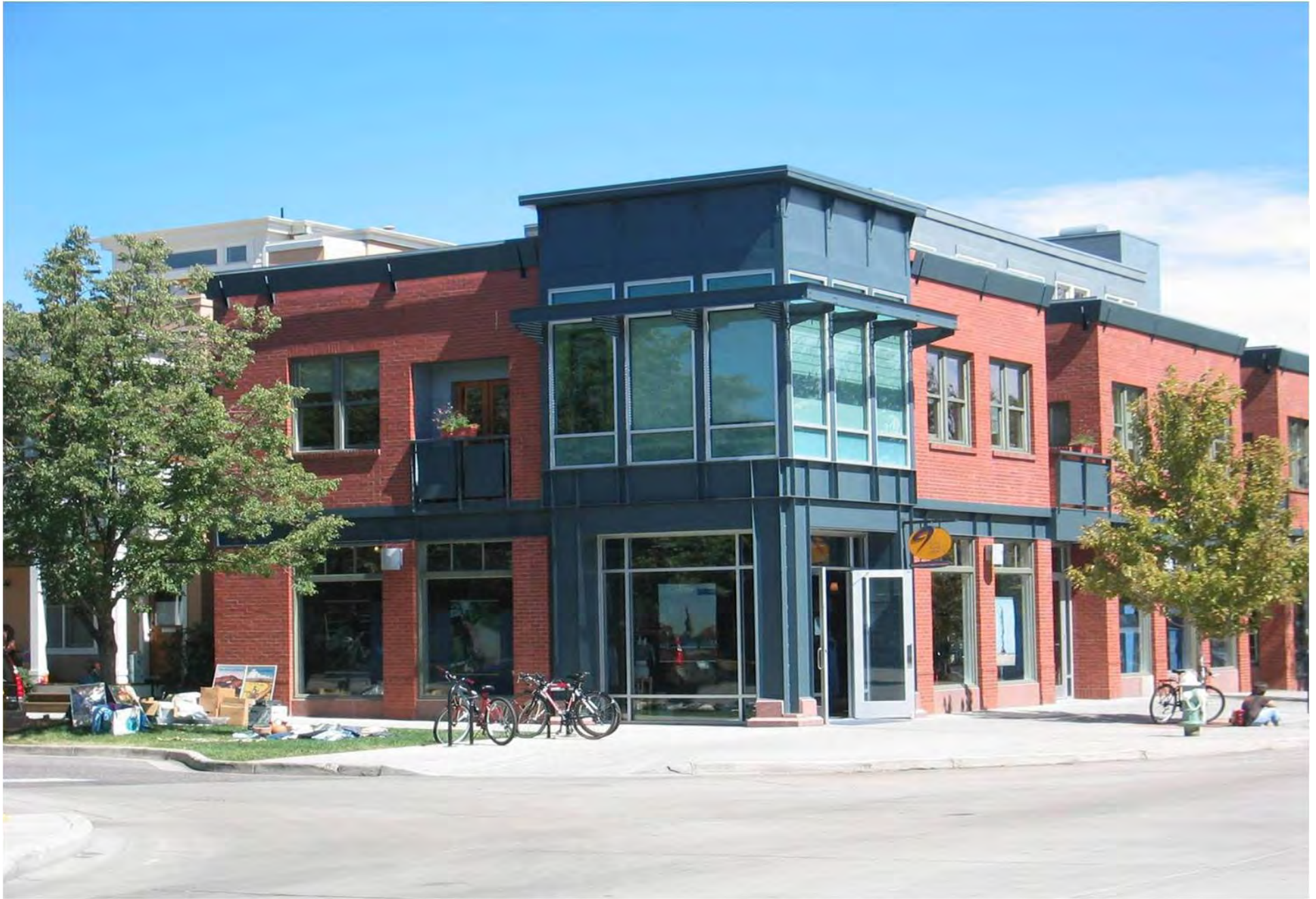
Figure 4.4 - Building with Visible Steel Support
