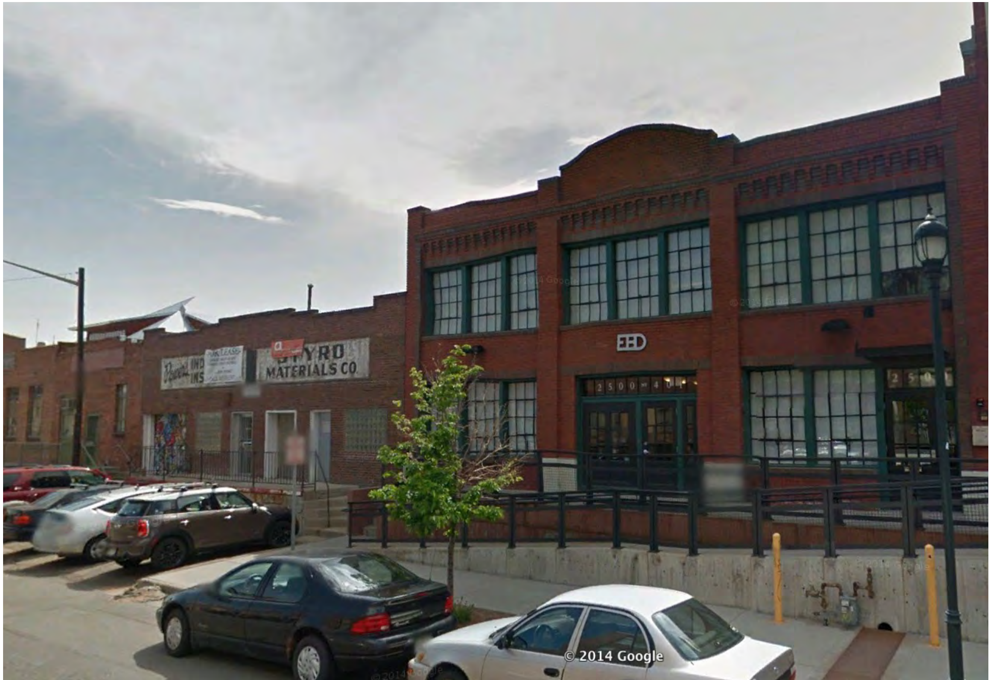
Figure 4.7 - Building with Multi-Paned Glass Windows
