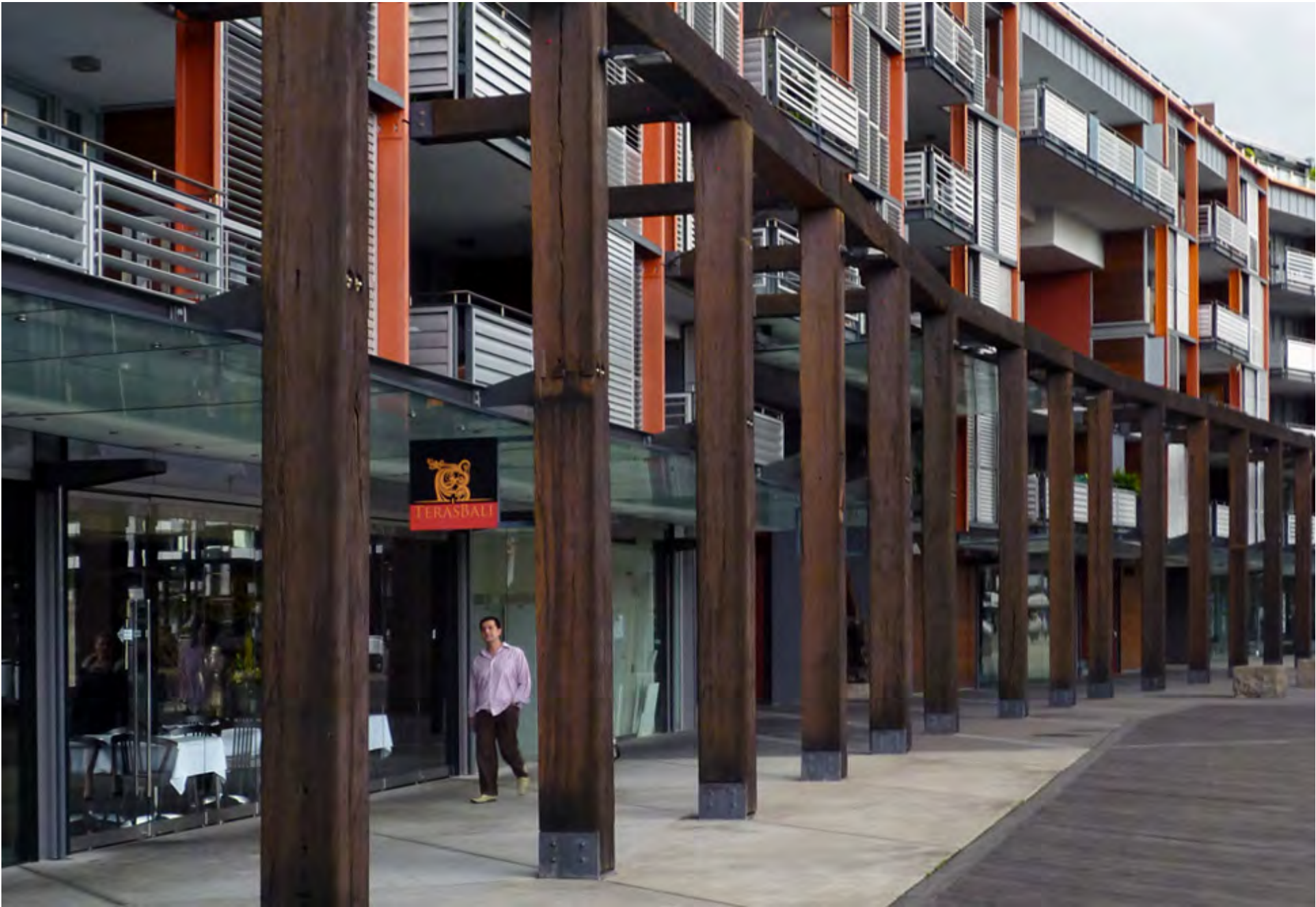
Figure 4.8 - Heavy Wood Timber Columns
