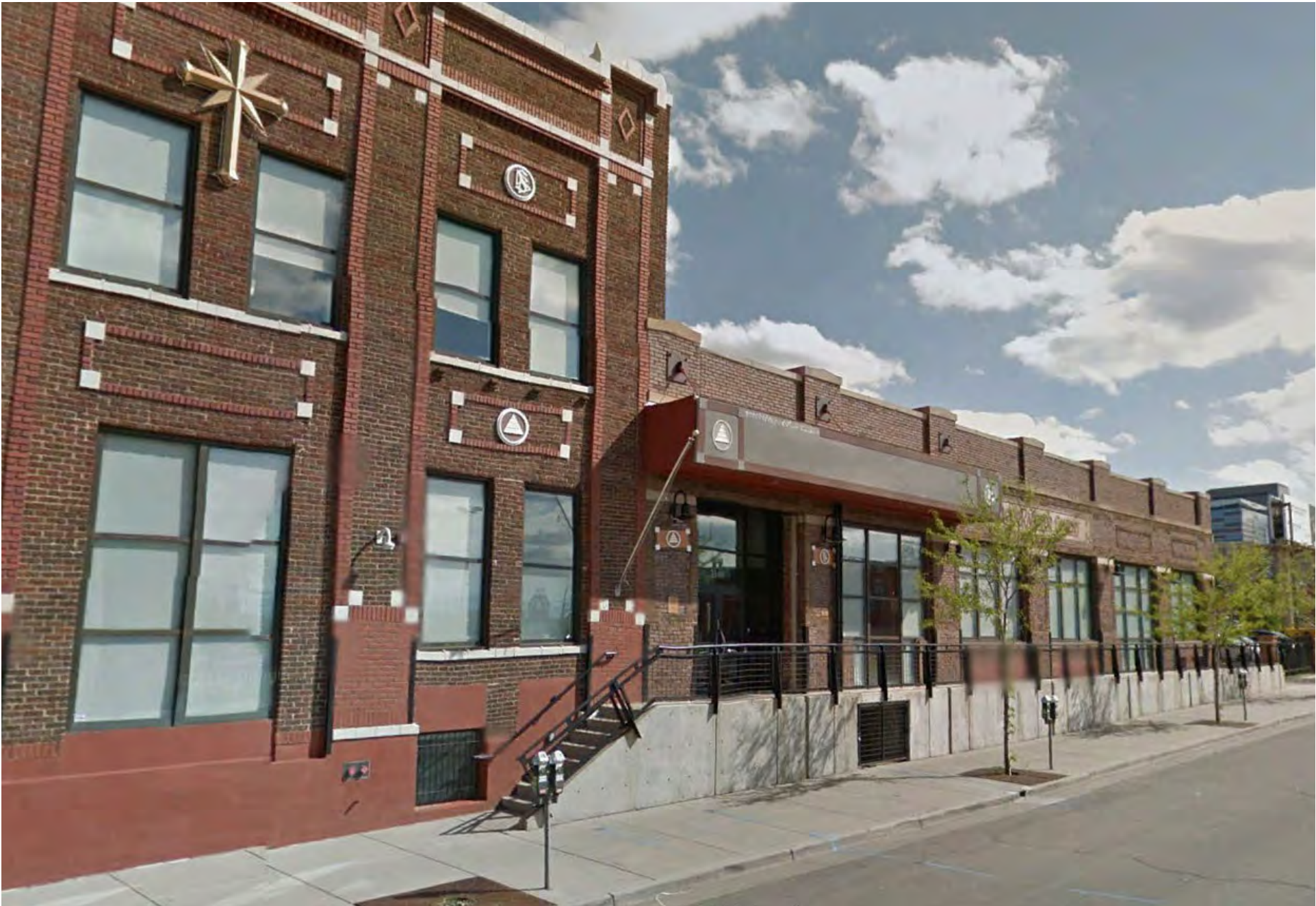
Figure 4.3 - Brick Building with Accent Banding
