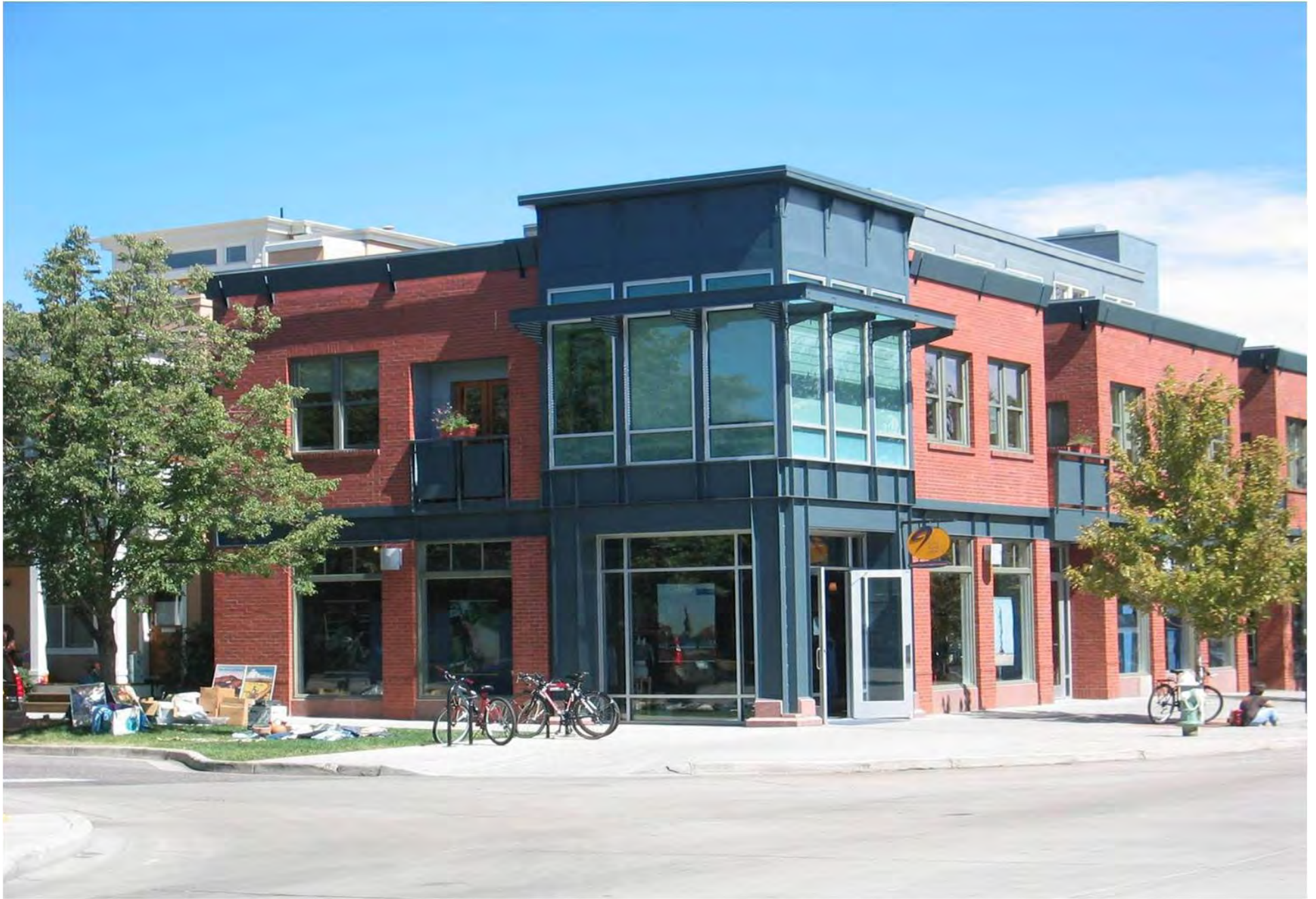
Figure 4.4 - Building with Visible Steel Support
