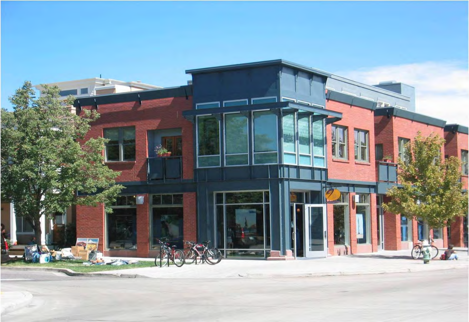
Figure 4.4 - Building with Visible Steel Support
