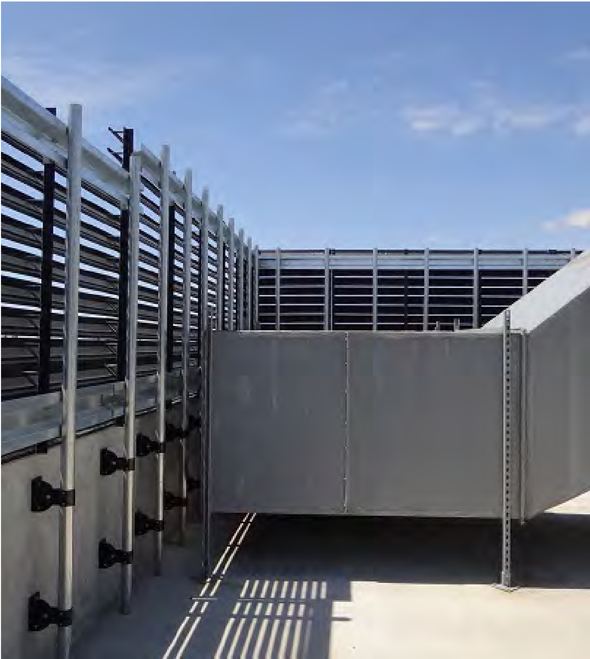
Figure 3.3 - Roof Equipment Screening
