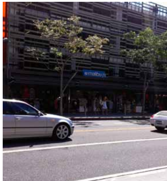
Figure 5.10 (1). Parking Structure Examples
