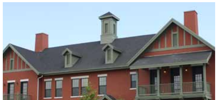
Roof Materials: Asphalt Composite Shingles
