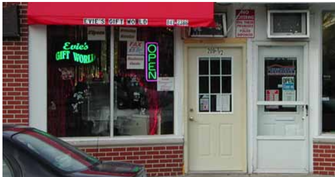
Prohibited: Residential Grade Doors on Commercial Buildings.
