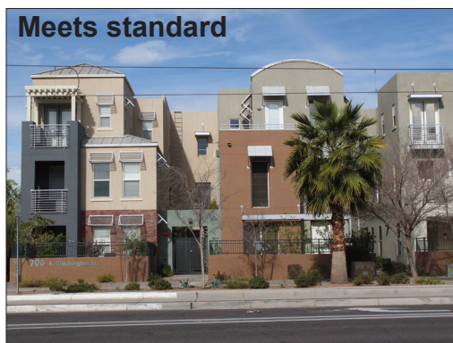
Figure 5.6.2.i and 5.6.2.j: Roofs should be simple in form, the building on the left does not meet this standard as the roof massing is overly complex while the building on the right has a more ordered variety in roof form.
