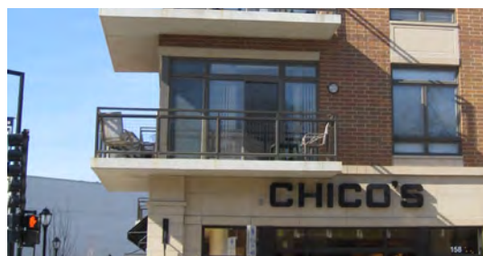
Figure 5.13 (5). Balconies Integral to Facade.
