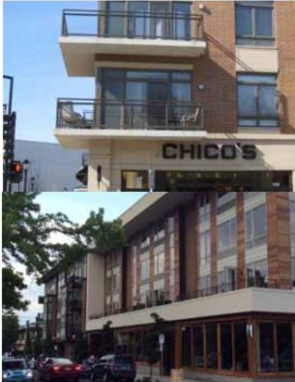
Figure: Balconies Integral to Facade
