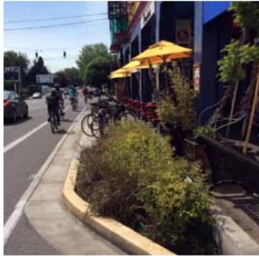
Figure: Curb Cut and Landscape Storm Drainage
