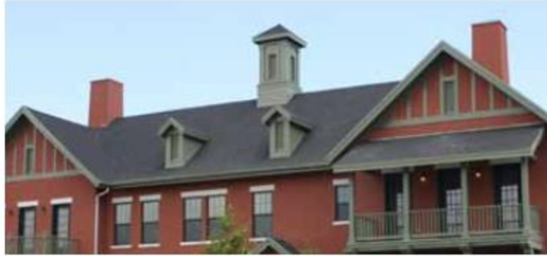
Roof Materials: Asphalt Composite Shingles
